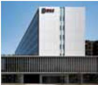
Headquarters / Engineering Research Center
