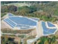
Mega-solar power business
